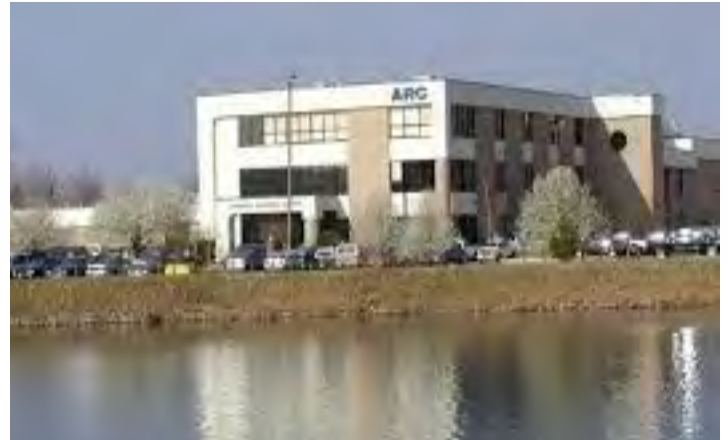
MDA ARC facility in Huntsville, AL. (Source: MDA )
